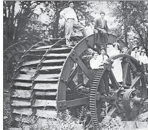
These early tourists stand on one of the large undershot wheels used to power the iron-making machinery.
