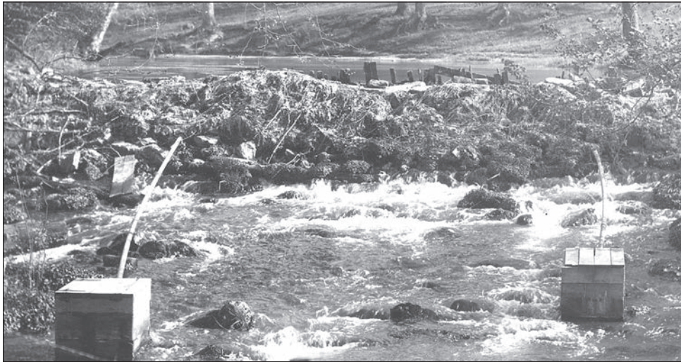
The dam at Maramec Spring, built in 1826, backs up water from the spring to create a pool of potential energy for the torrent of the spring branch.
