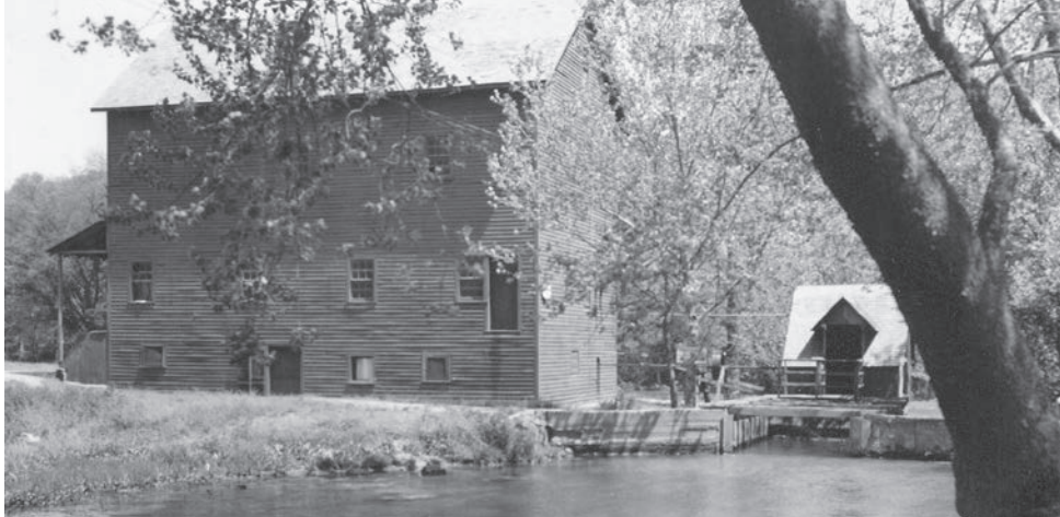
Four flour and grist mills were constructed to utilize the power of Bennett Spring to process grains. Above is the fourth mill which stood until 1944.
